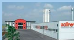
Company buildings ShopCrea wallner. Firmengebäude ShopCrea wallner.
