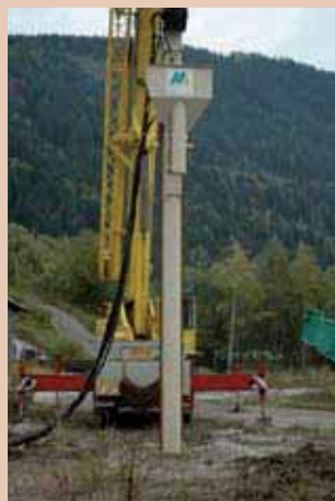
Vibrolance with bottom feed. Schleusenrüttler.
