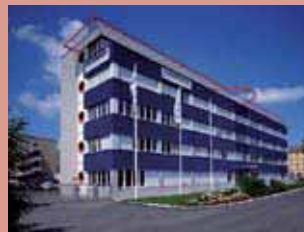
Schrack Seconet Headquarters Vienna. Schrack Seconet Headquarter Wien
